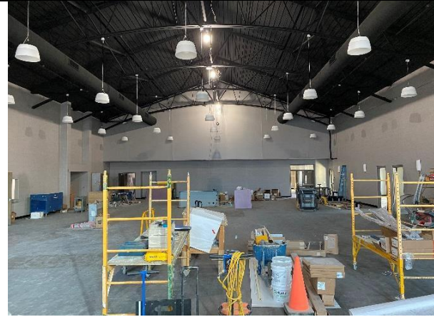
Fellowship Hall facing East
