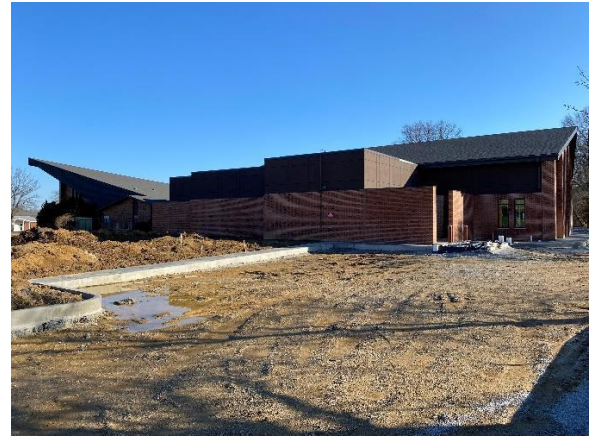
View from North
