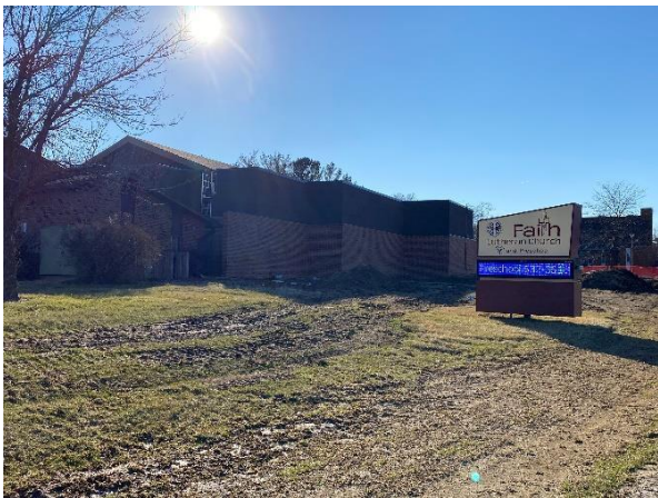
North Site Work
