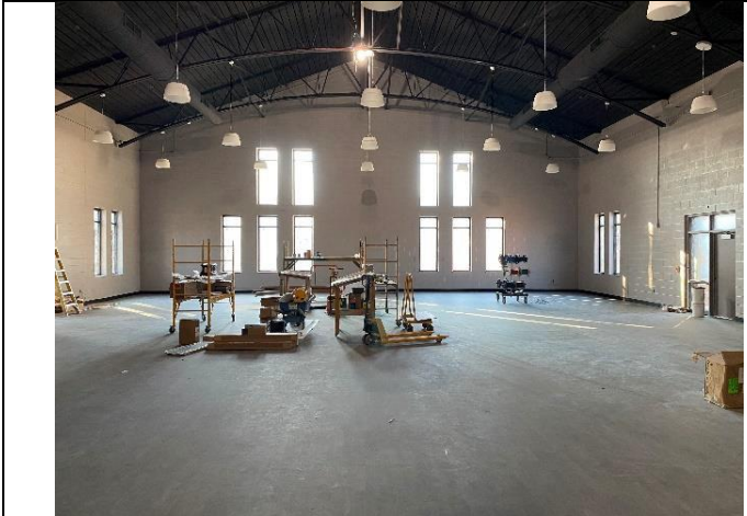
Fellowship Hall facing West
